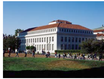
U.C. Berkeley Bancroft Special Collections Library Renovation
